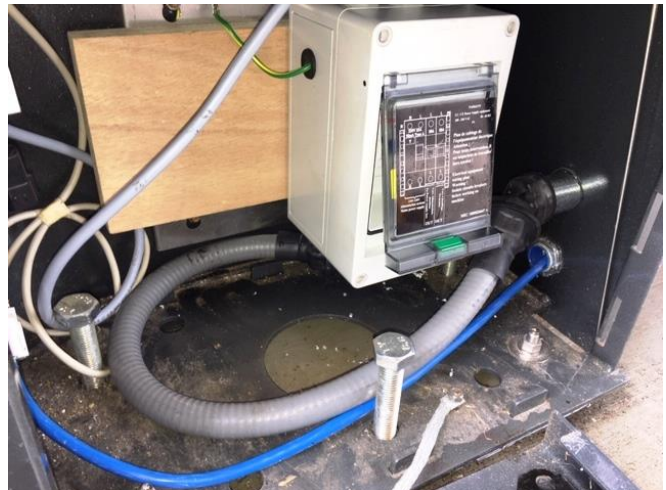
Photo 8- Client Added Seal-Tite Protection
