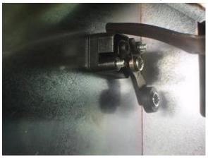
B. Place a flat head screwdriver behind the collection switch; slowly and carefully pry the collection off of the studs by turning the screwdriver from side to side.
